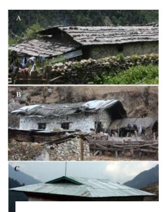
Figure 2 Types of roofing materials used in the study area (A)Shingles (B) Bamboo mats [Conventional] & (C) CGI sheets.
